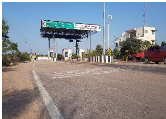
Toll Plaza and Building at Km. 12+000
