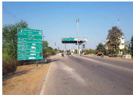
Toll Plaza at Km. 75+900
