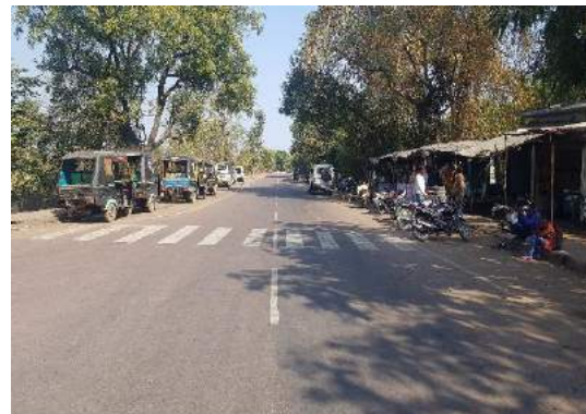
Pedestrian Markings at Km. 48+200
