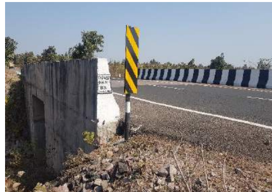
Road safety at Box Culvert at Km. 24+637
