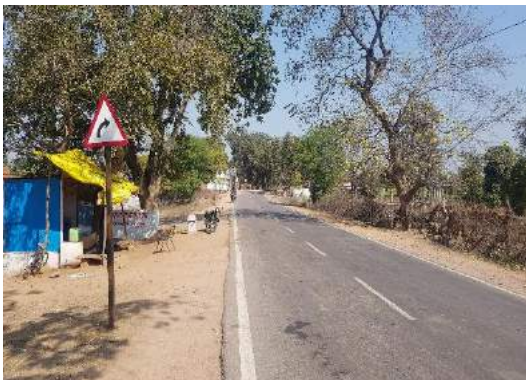
Curve Ahead sign board at Km. 48+000
